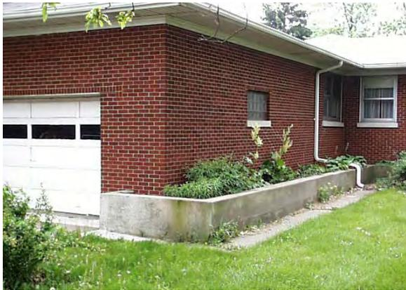
This Calumet City home is surrounded by a floodwall, but the garage door must be sandbagged during a flood. The wall doubles as a planter box to reduce the visual impact of a flood protection structure.
