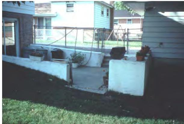
This floodwall was installed by a South Holland homeowner on the Calumet Union Drainage Ditch. It has kept floodwaters out of the house multiple times since it was built in 1991.
